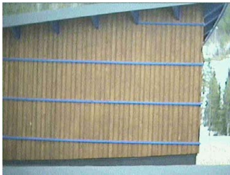
A tower part on the roof (Sports hall)
