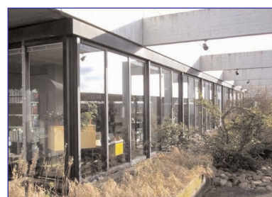
Figure 7: Exterior view of offices on the roof terrace
