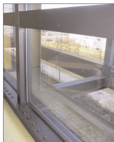
Figure 5: Air curtain outlet at bottom of window
