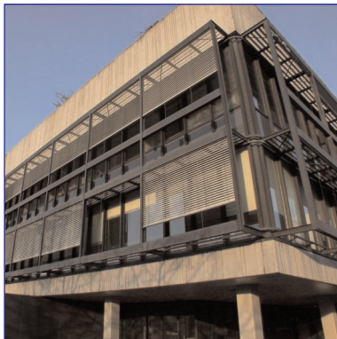
Figure 4: Facade detail showing the shading systems
