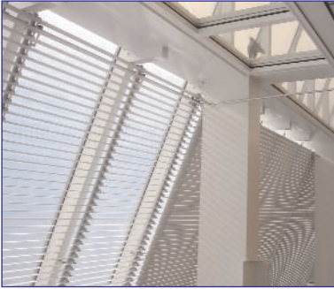
Figure 4: Controlable blinds ensure comfortable inside temperatures
