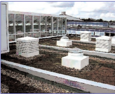
Figure 5: The sedum roof with the sun pipes and passive ventilation units
