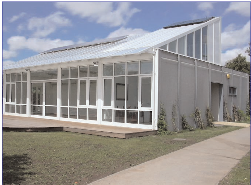
Figure 6: One classroom has cedar cladding, this classroom has weldmesh for plants to grow up the walls
